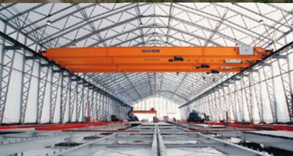
Giebelhallen (15m - 80m)
